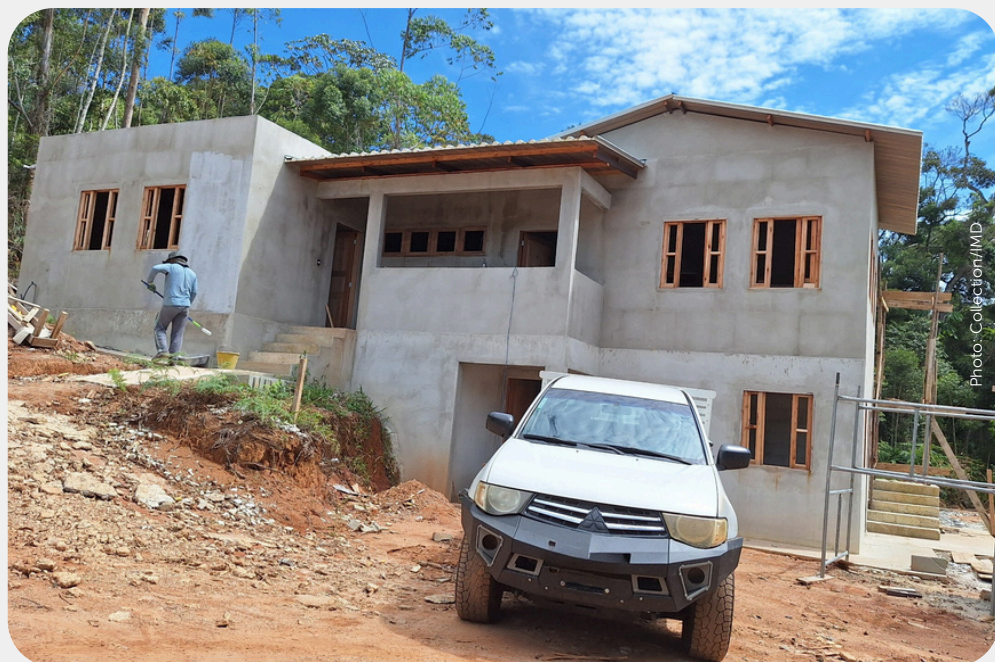
Finishing work on the research center at the Kaetés Reserve.
