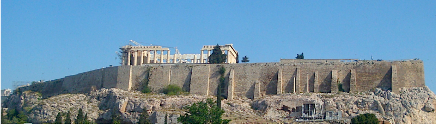
Though covered with scaffolding, the Parthenon and the hulking mass of the Acropolis still impresses. (Photo by guide Megan Crewe)
